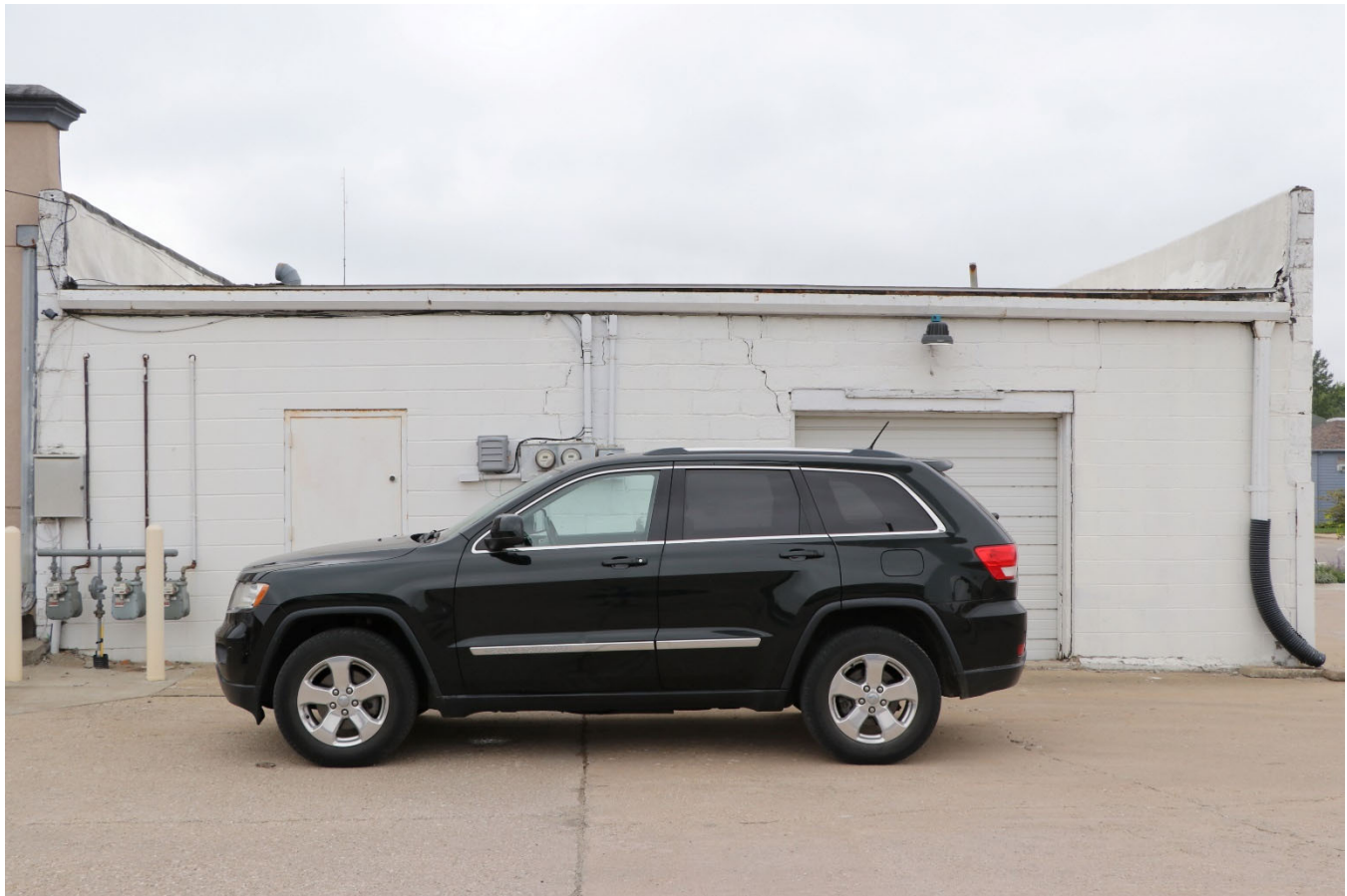
Photograph 44-00447-005. North elevation, looking south (October 2023)
