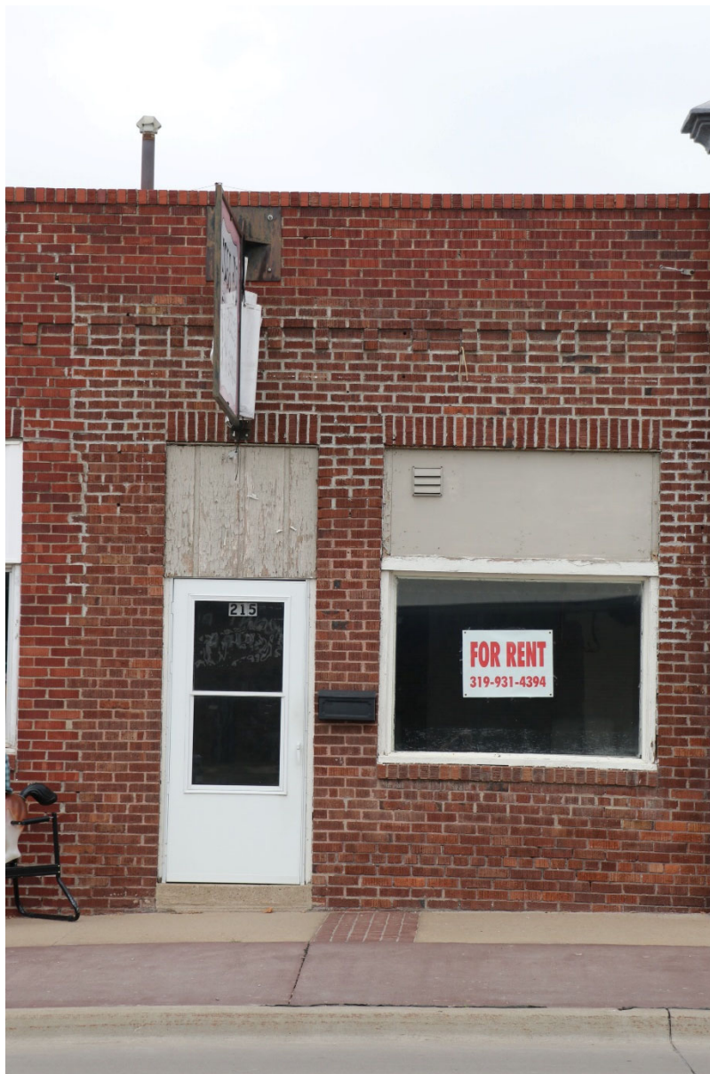
Photograph 44-00447-003. East half of south elevation, looking north (October 2023)
