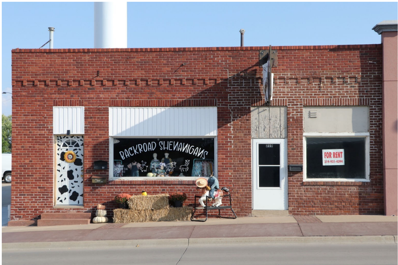
Photograph 44-00447-001. South elevation, looking north (October 2023)
