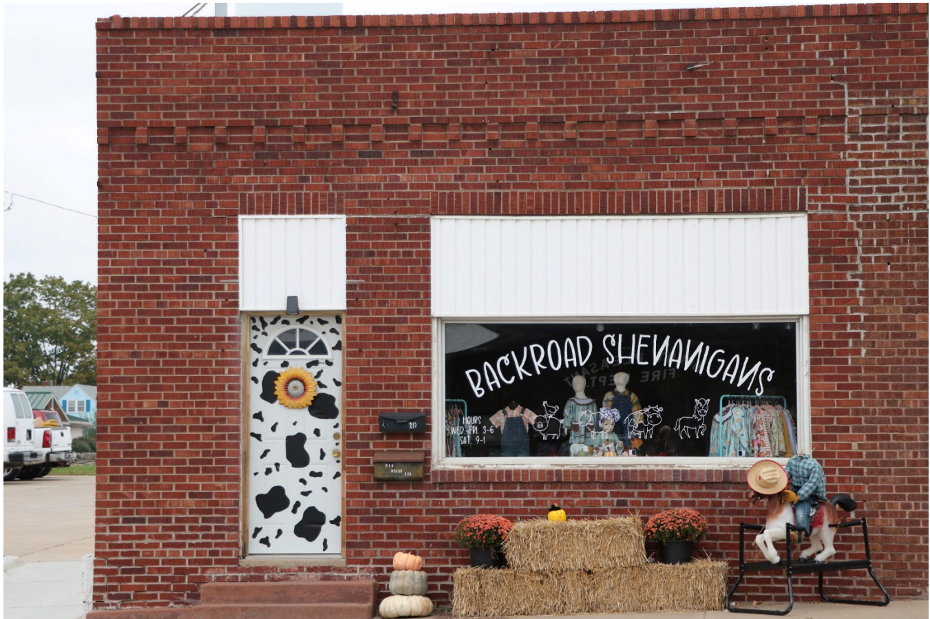
Photograph 44-00447-002. West half of south elevation, looking north (October 2023)
