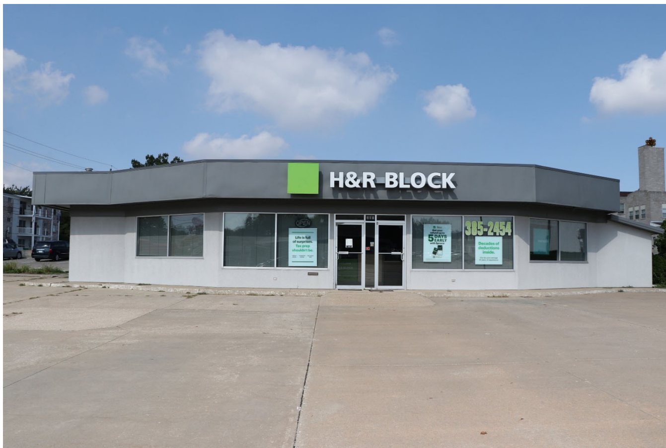
Photograph 44-02277-001. South elevation, looking north (October 2023)
