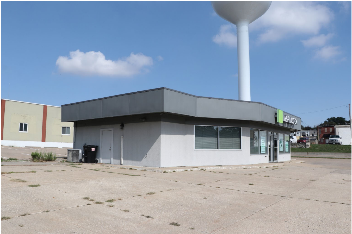
Photograph 44-02277-002. West and south elevation, looking northeast (October 2023)
