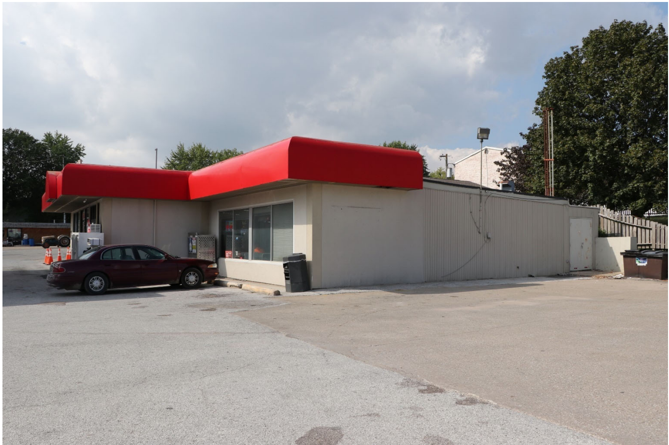
Photograph 44-02278-002. East elevation, looking northwest (October 2023)
