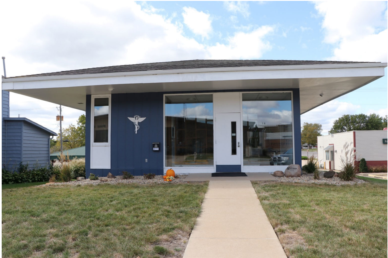
Photograph 44-02240-001. East elevation, looking west (October 2023)
