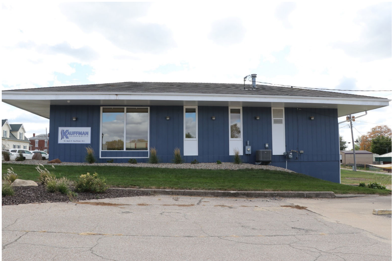
Photograph 44-02240-002. North elevation, looking south (October 2023)
