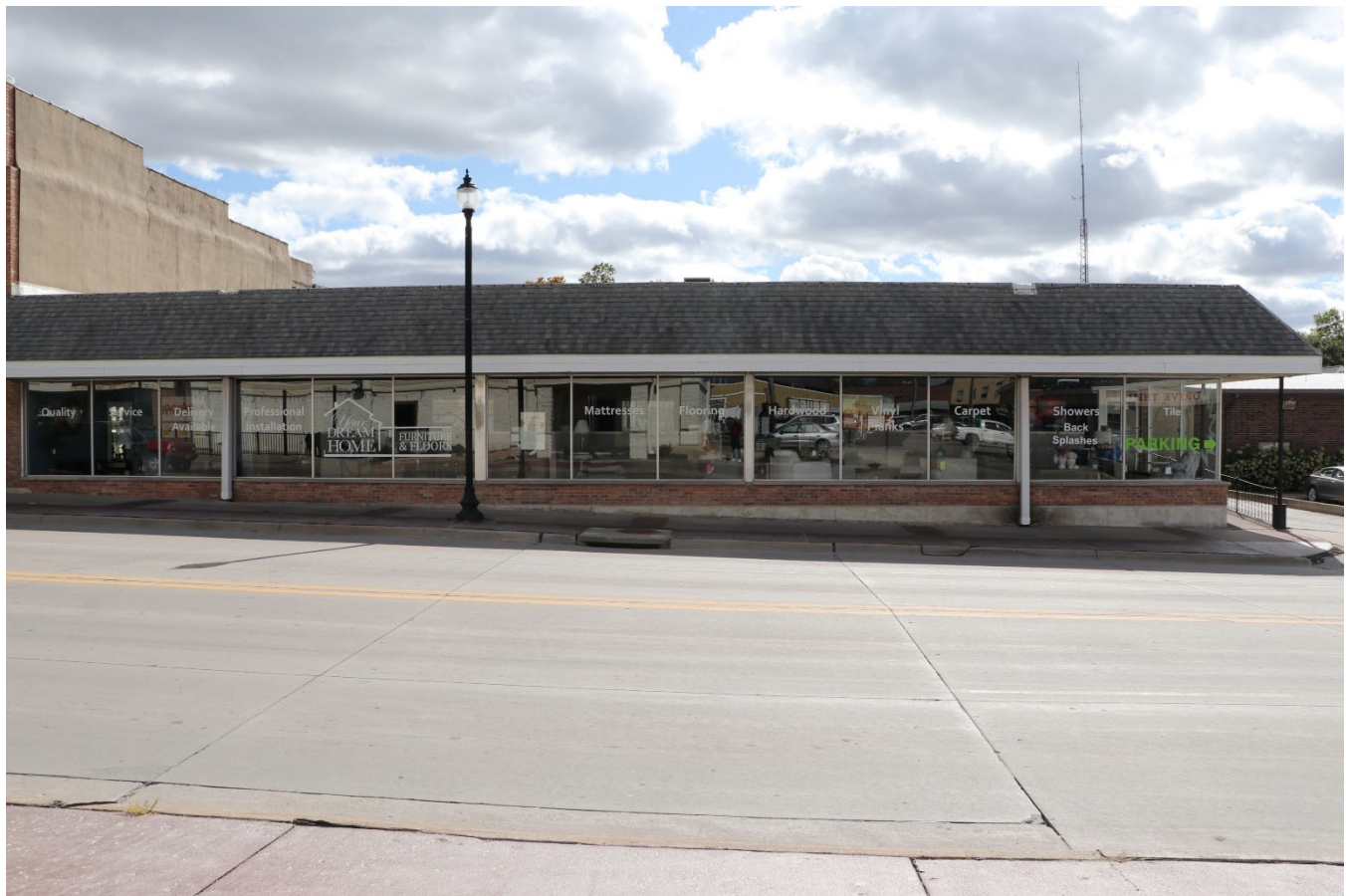
Photograph 44-00445-001. North elevation, looking south (October 2023)
