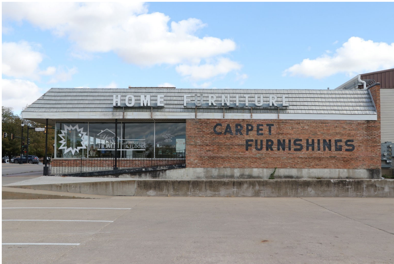
Photograph 44-00445-002. West elevation, looking east (October 2023)
