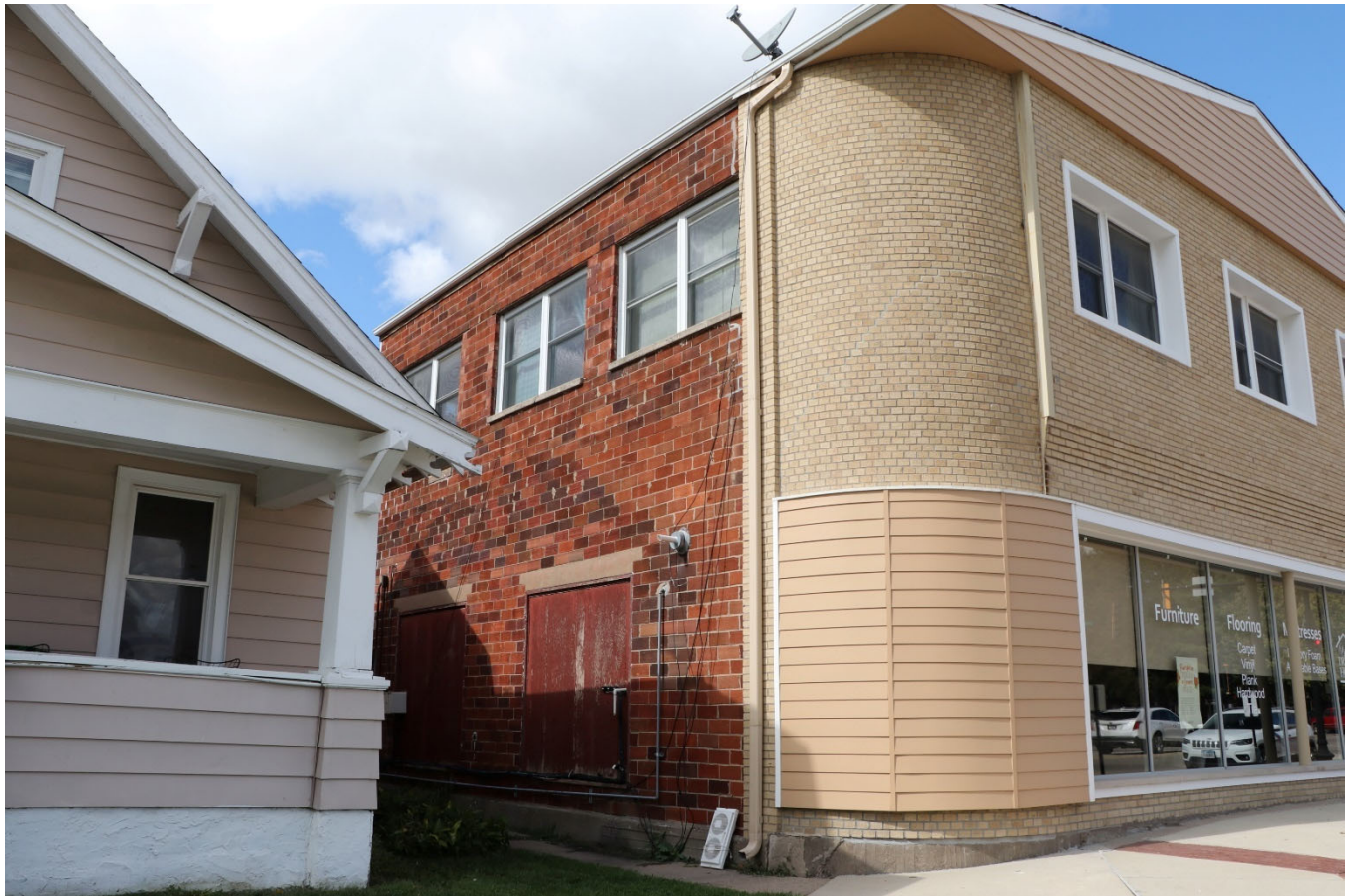
Photograph 44-02251-002. South elevation, looking northwest (October 2023)
