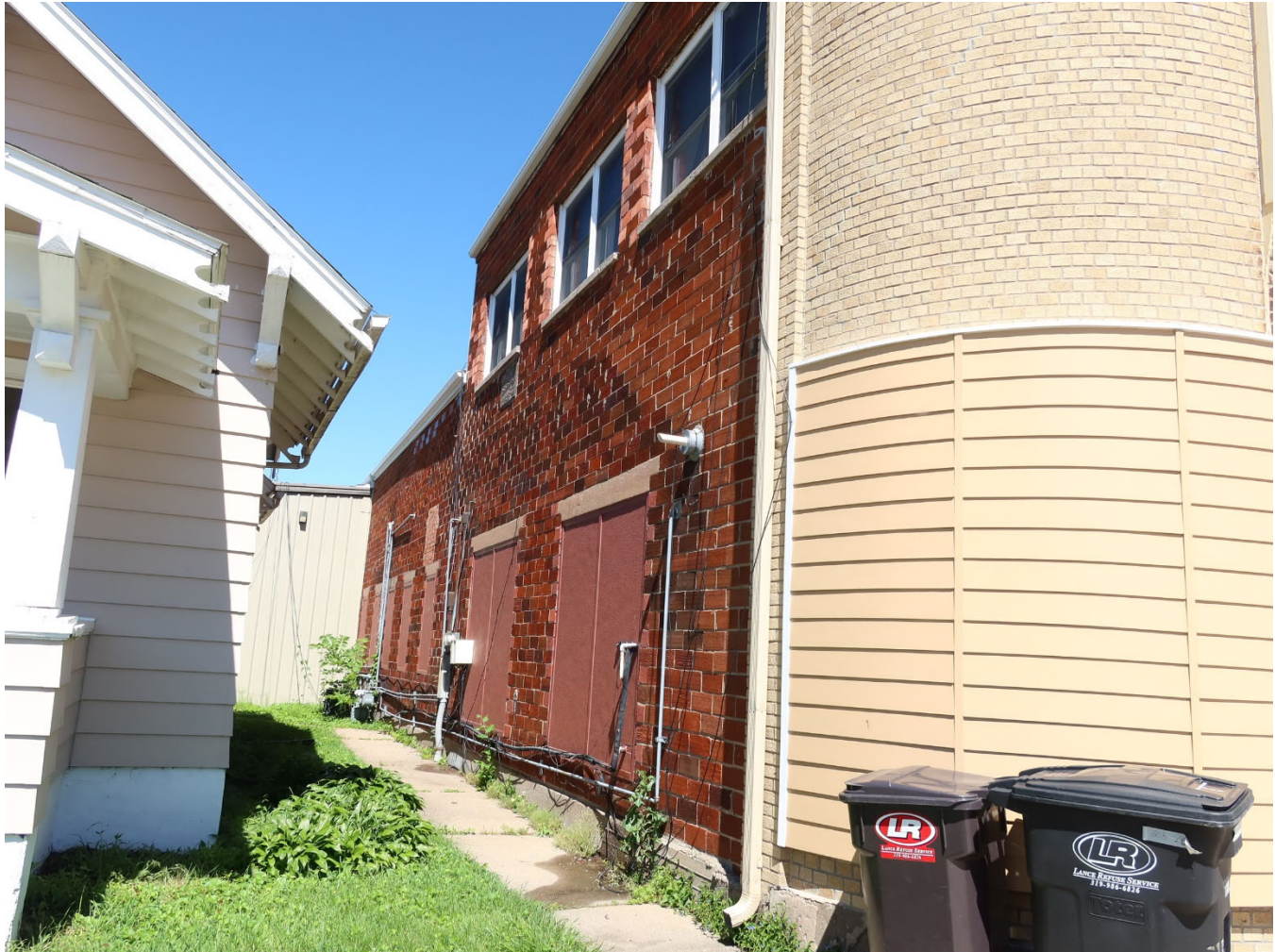
Photograph 44-02251-003. South elevation, looking northwest (June 2024)
