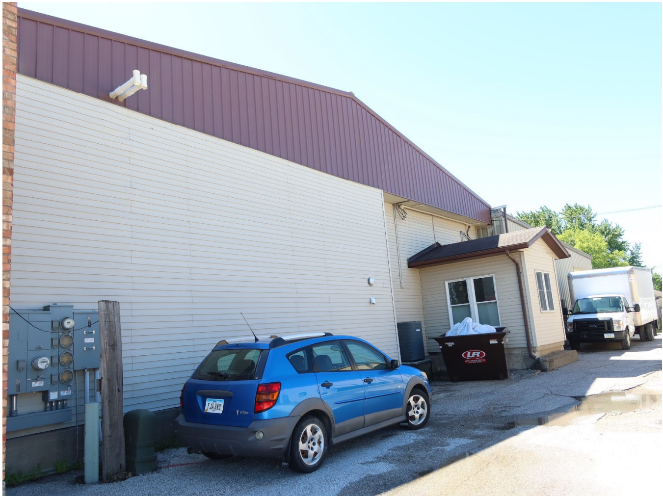
Photograph 44-02251-004. West elevation, looking southeast (June 2024)
