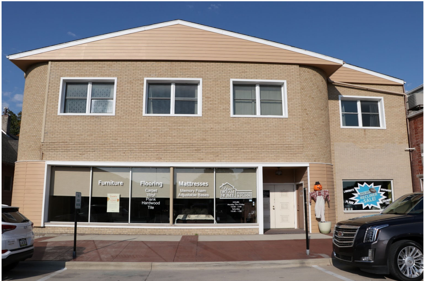
Photograph 44-02251-001. Façade of building, looking west (October 2023)
