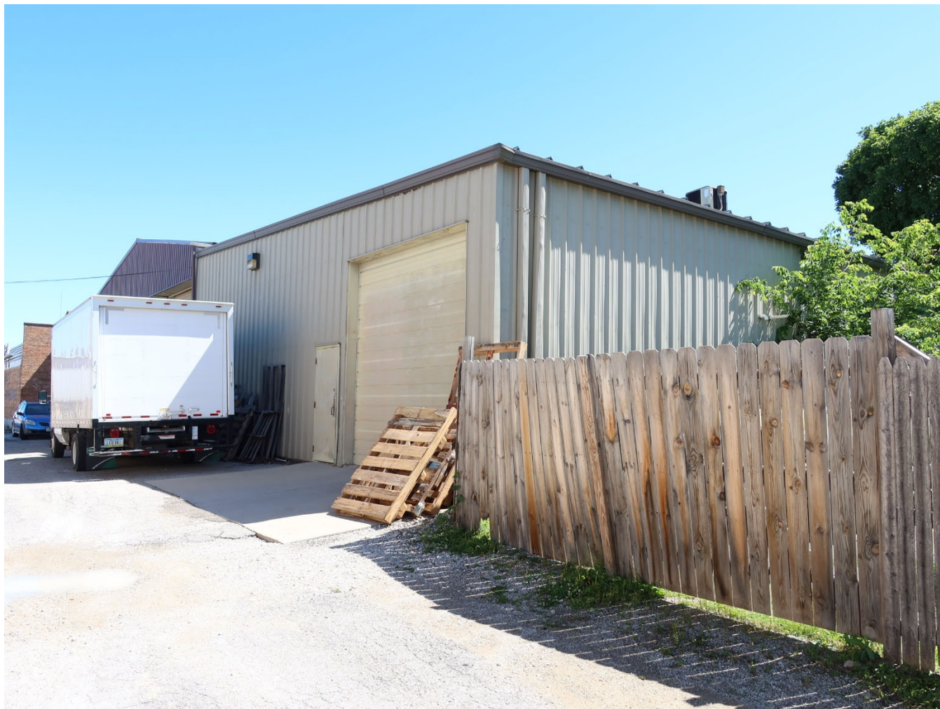
Photograph 44-02251-005. West elevation, looking northeast (June 2024)
