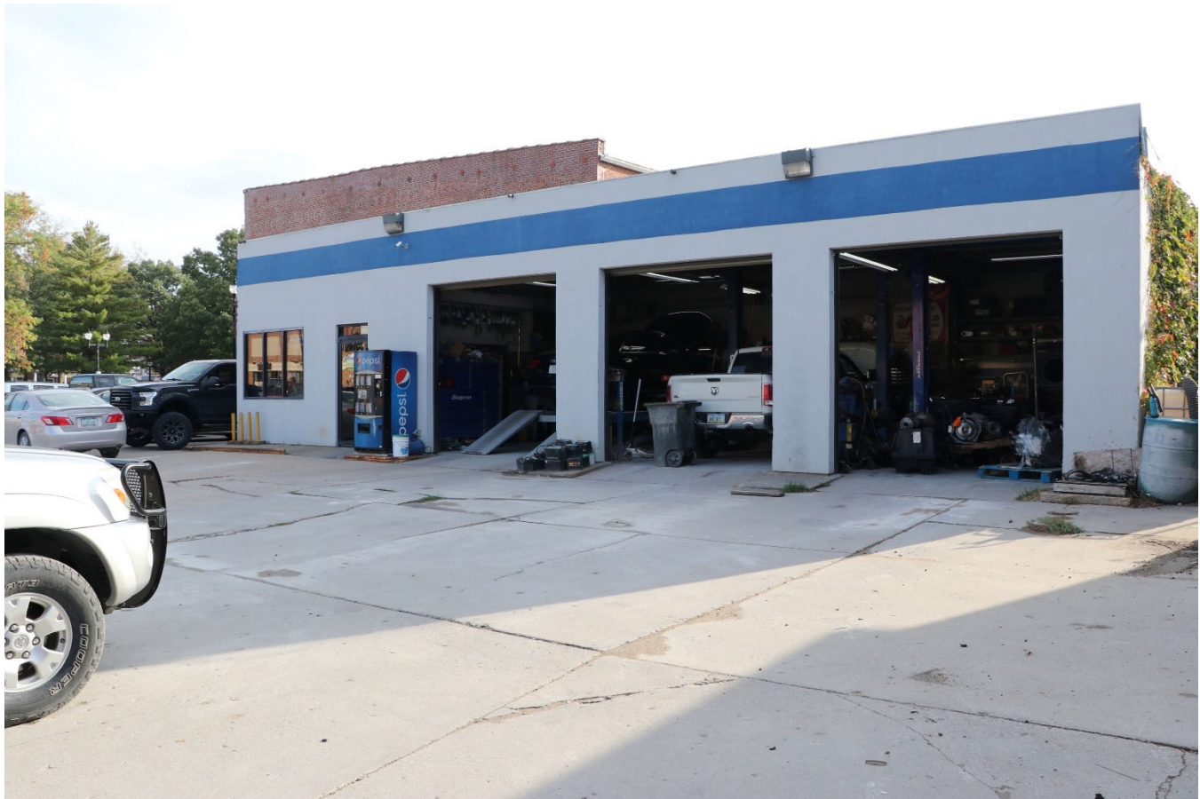
Photograph 44-00413-001. West elevation, looking northeast (October 2023)
