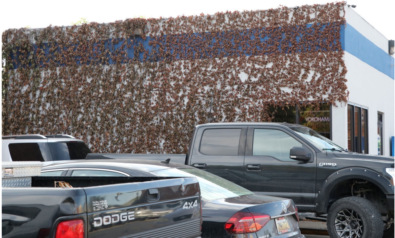
Photograph 44-00413-002. North elevation, looking south (October 2023)
