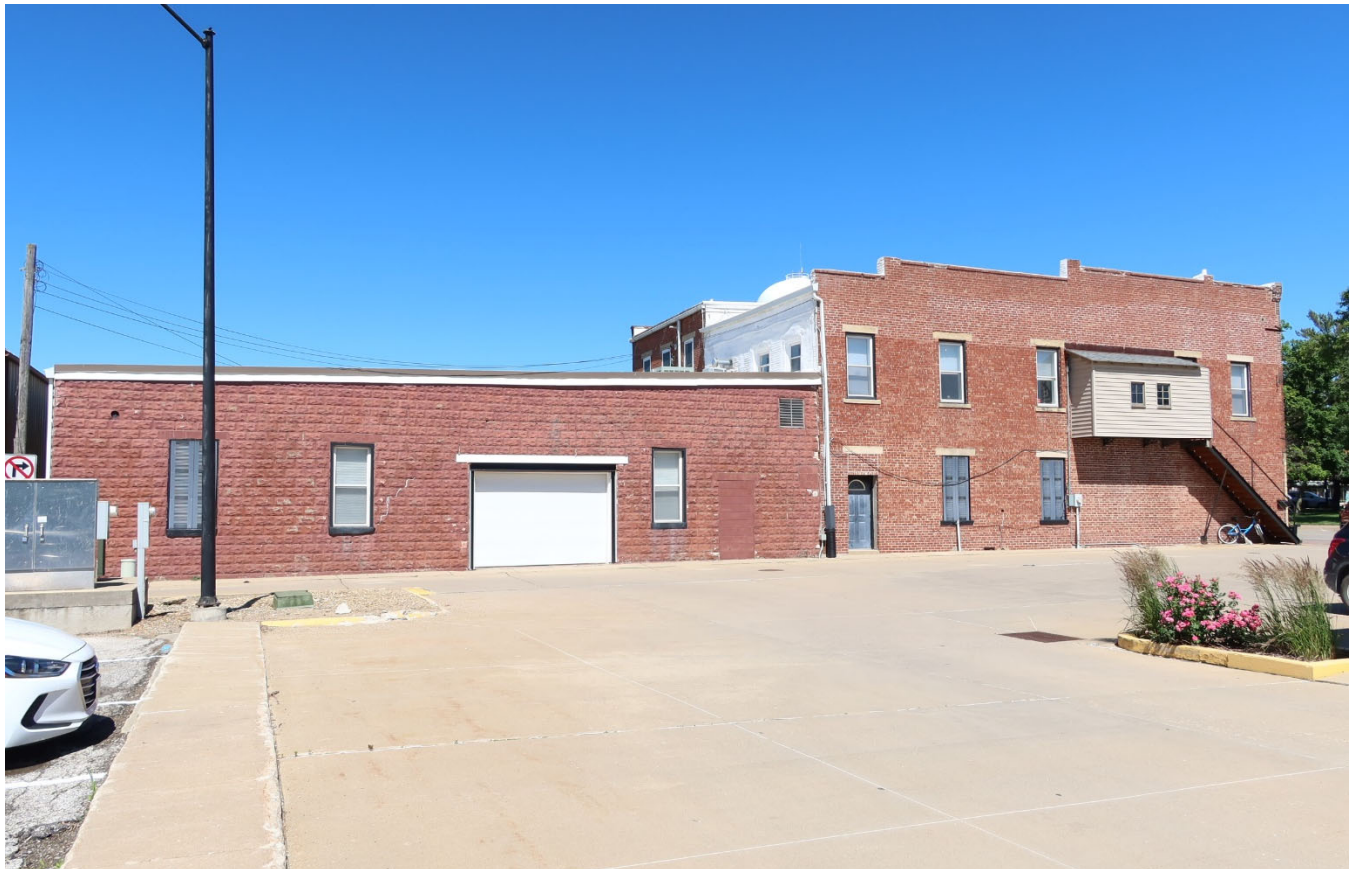
Photograph 44-00443-003. East elevation, looking west (June 2024)
