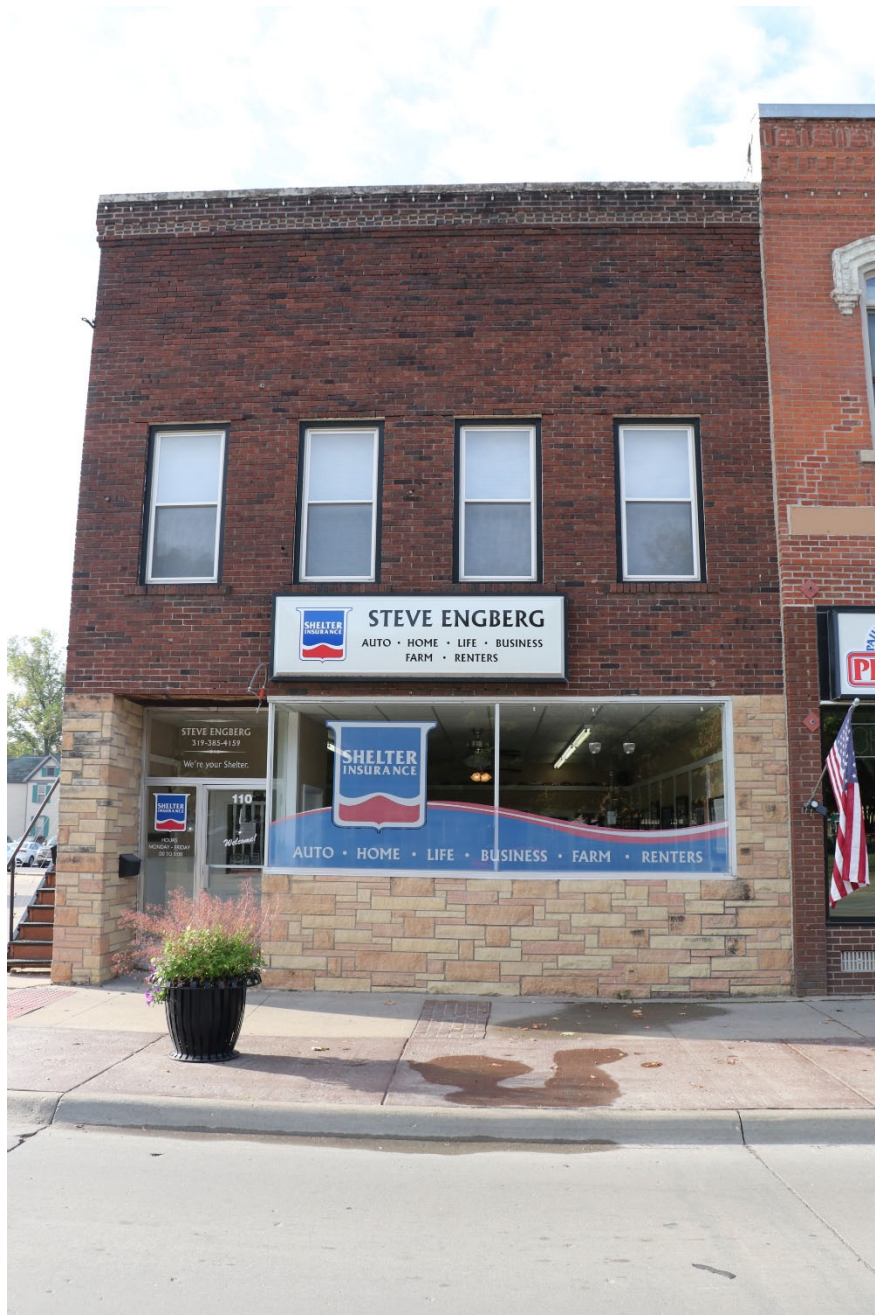
Photograph 44-00443-001. Façade of building, looking south (October 2023)
