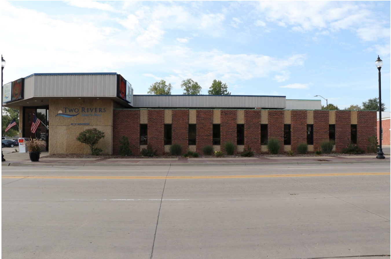
Photograph 44-00441-002. North elevation, looking south (October 2023)
