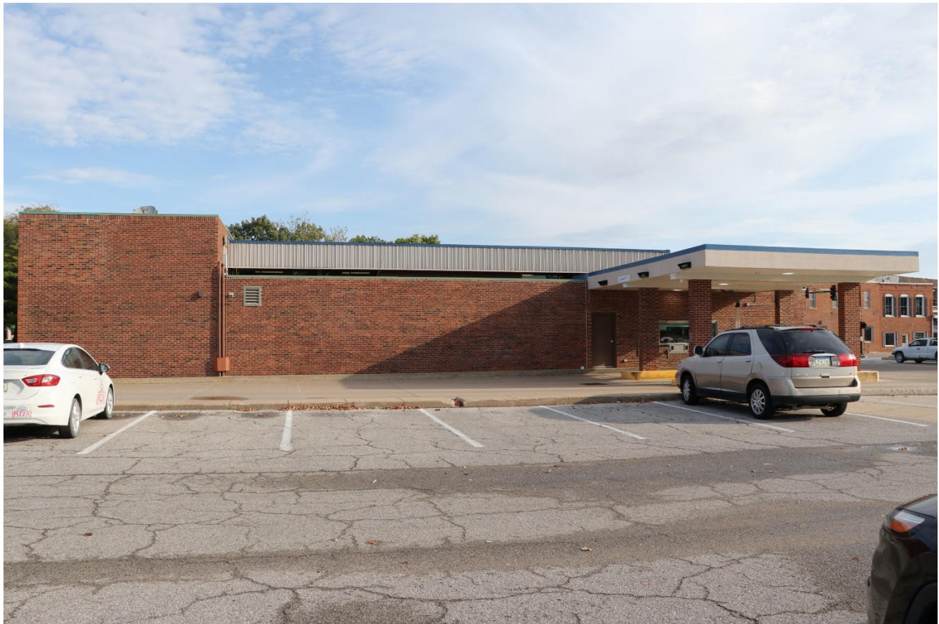
Photograph 44-00441-005. South elevation, looking north (October 2023)
