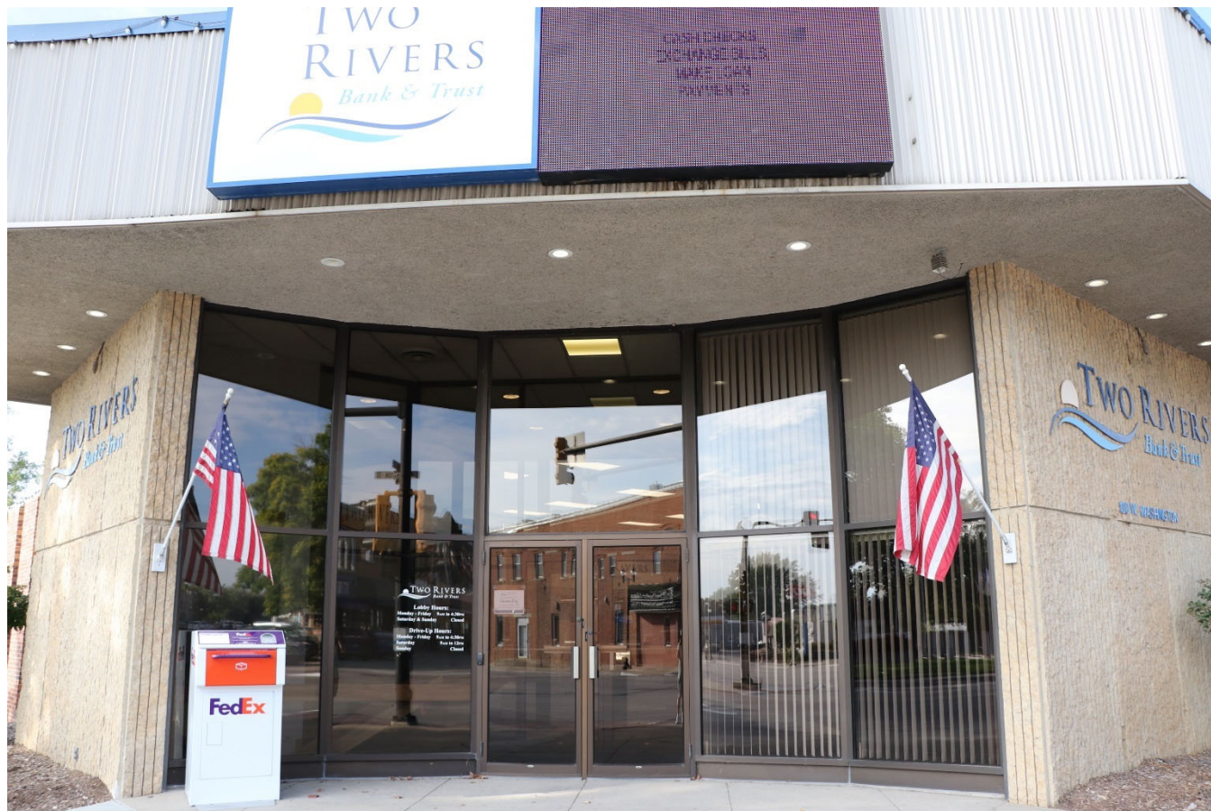
Photograph 44-00441-003. Entry to building, looking southwest (October 2023)
