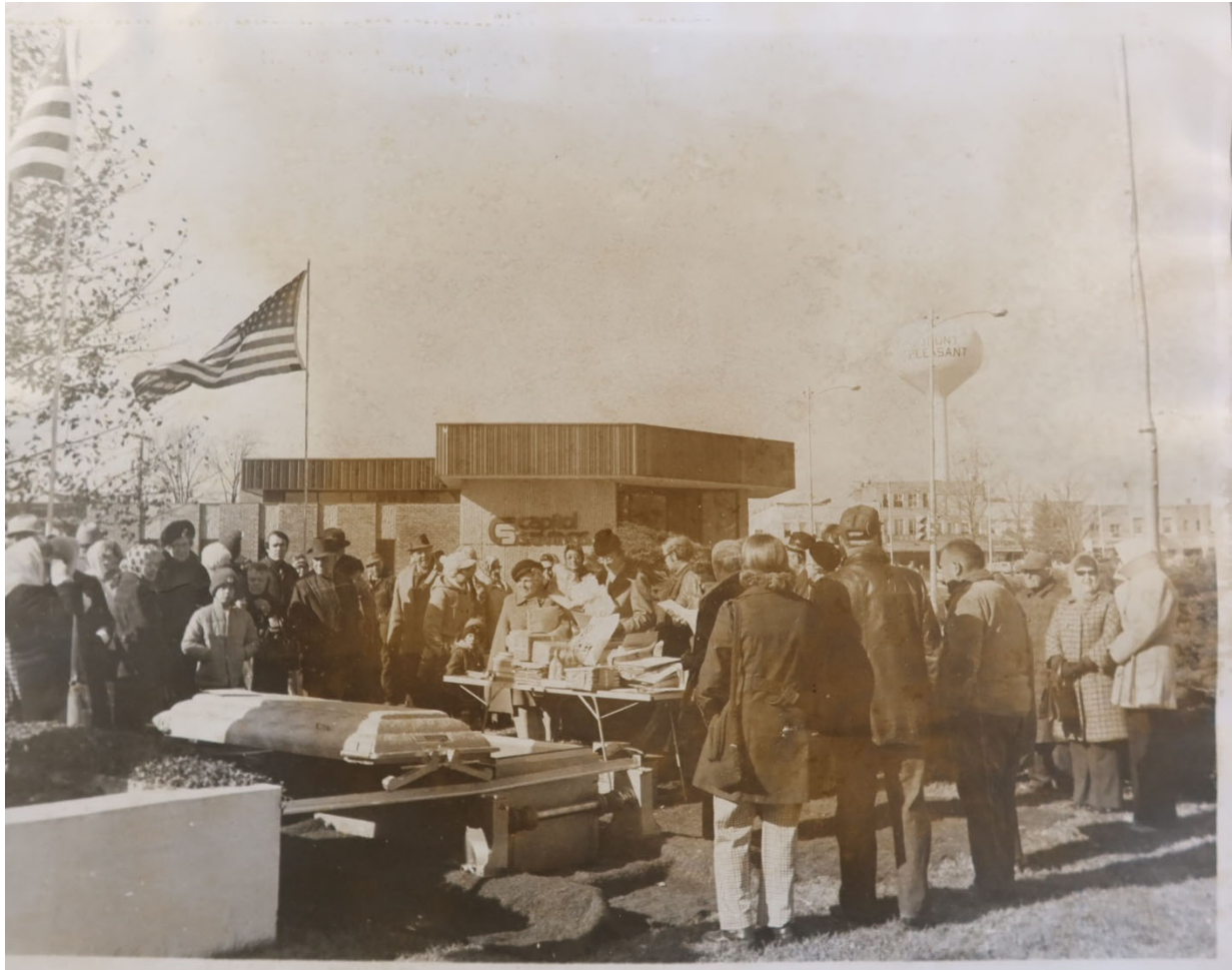
East elevation of building from courthouse block, looking west (1976 bicentennial capsule ceremony, HCHS, Mt Pleasant library binder)
