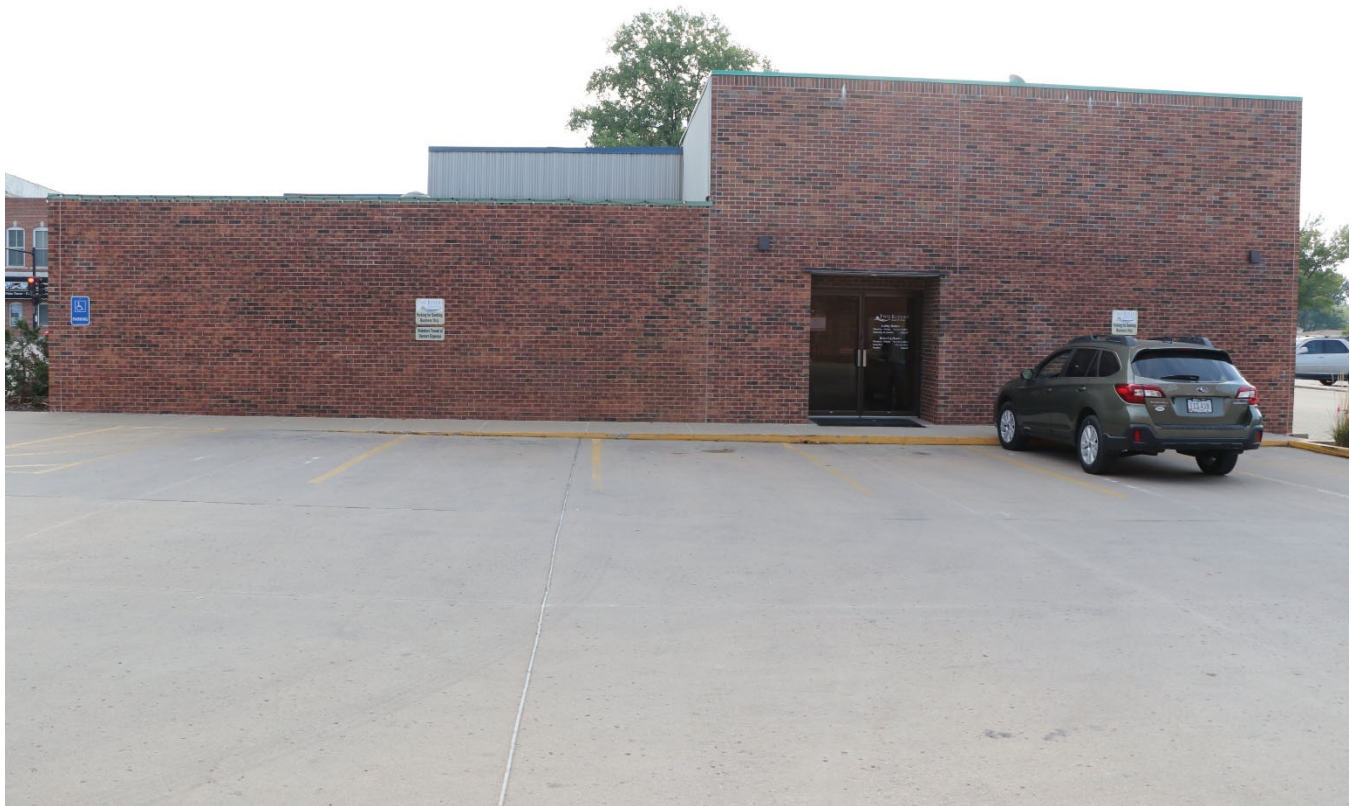
Photograph 44-00441-004. West elevation, looking east (October 2023)
