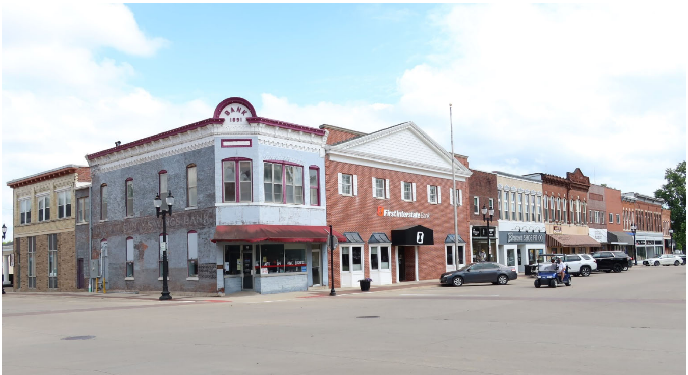
Photograph 44-02280-028. East side of 100 block of S. Main St (DT-110-120), looking southeast
