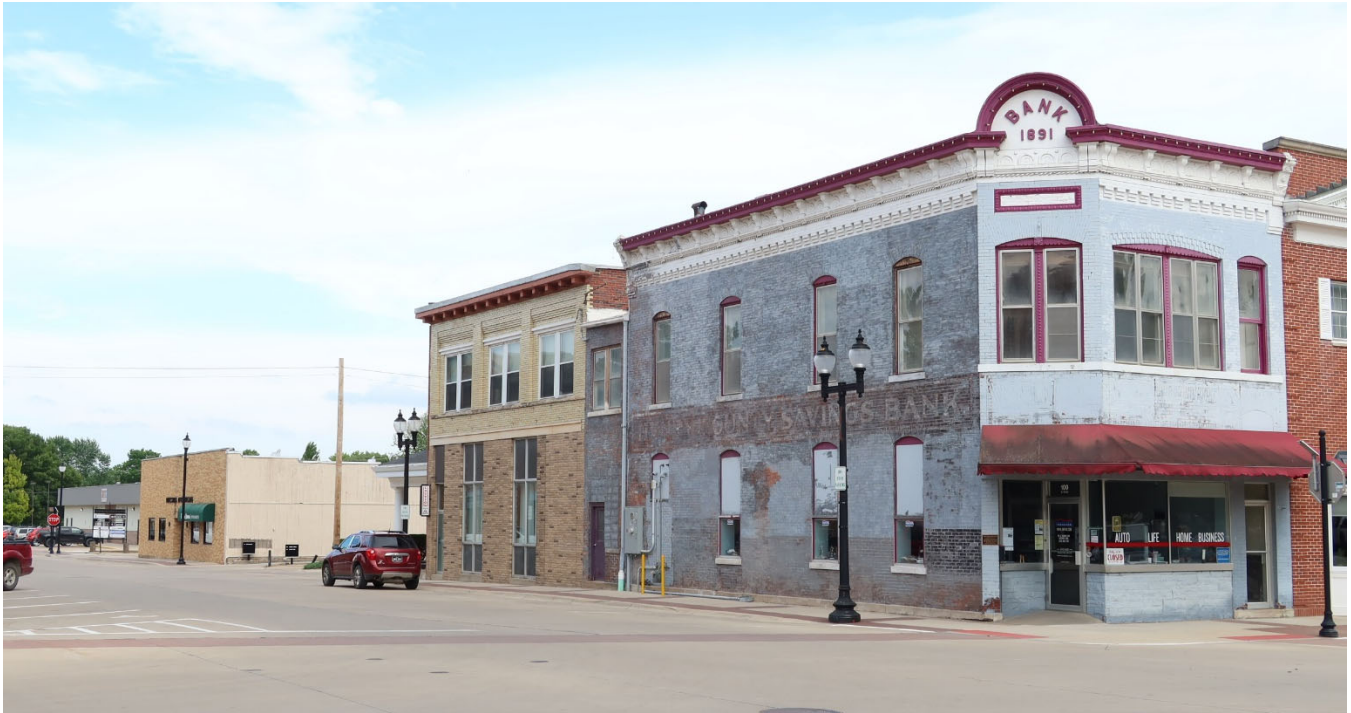
Photograph 44-02280-027. South side of 100 block of E. Monroe St (DT-109-111), looking southeast
