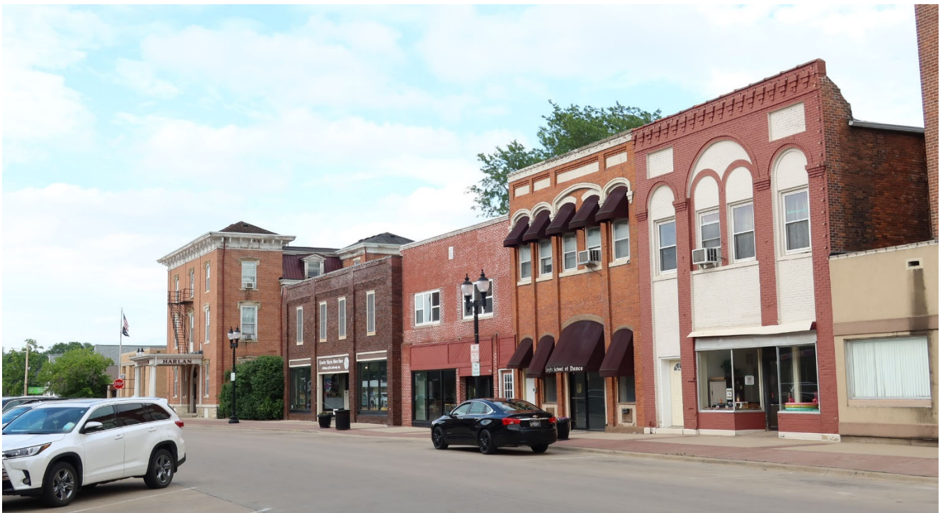
Photograph 44-02280-014. East side of 100 block of N. Jefferson St (DT-60-65), looking northeast
