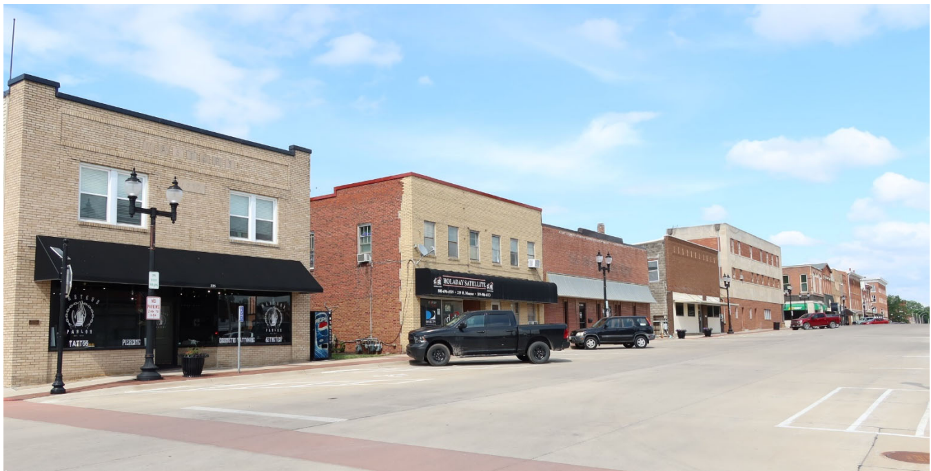
Photograph 44-02280-008. North side of 200 block of W. Monroe St (DT-32-36), looking northeast
