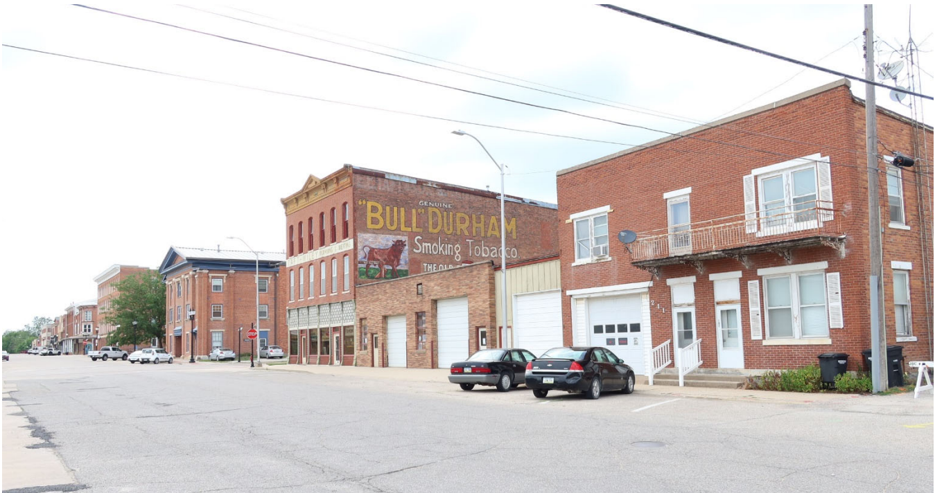
Photograph 44-02280-024. North side of 100-200 block of E. Monroe St (DT-102-106), looking northwest
