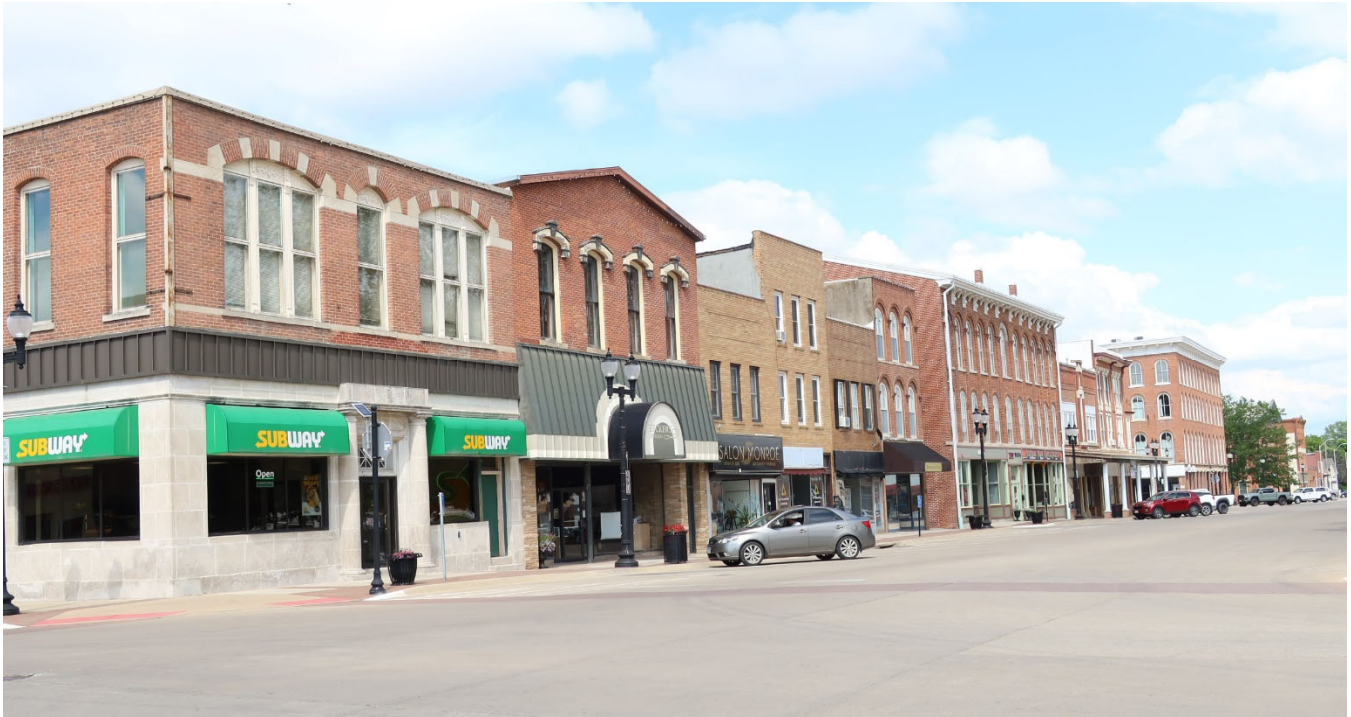
Photograph 44-02280-015. North side of 100 block of W. Monroe St (DT-65-73), looking northeast
