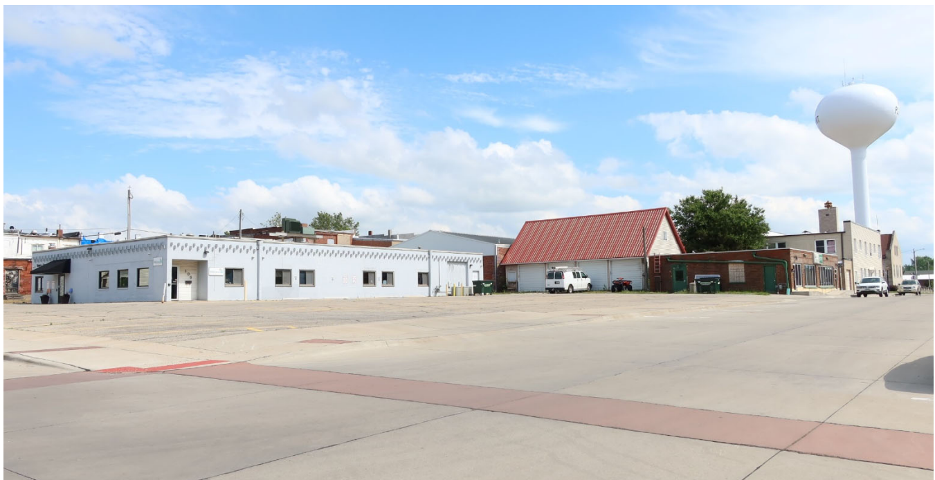
Photograph 44-02280-010. East side of 100 block N. Jackson St (DT-30-32), looking southeast
