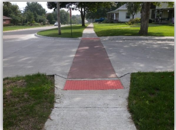
Modern crosswalk with ADA accessible curb ramps and warning tiles— Main and Green Streets
